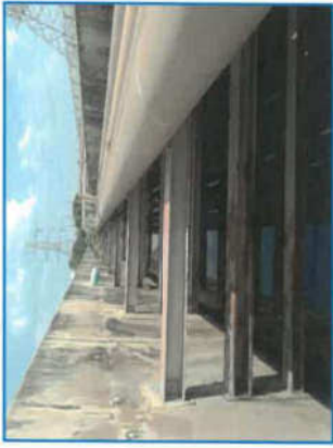
Picture 1 Visual inspection support and suspension found corrosion
