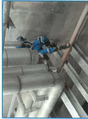
Picture 2 Measurement thickness pipe fuel oil system
