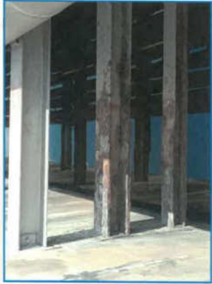
Picture 1 Visual inspection support and suspension found corrosion
